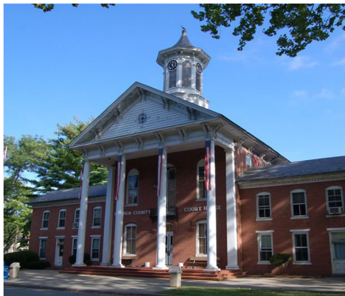
The Warren County Courthouse in Belvidere as it appears today.
