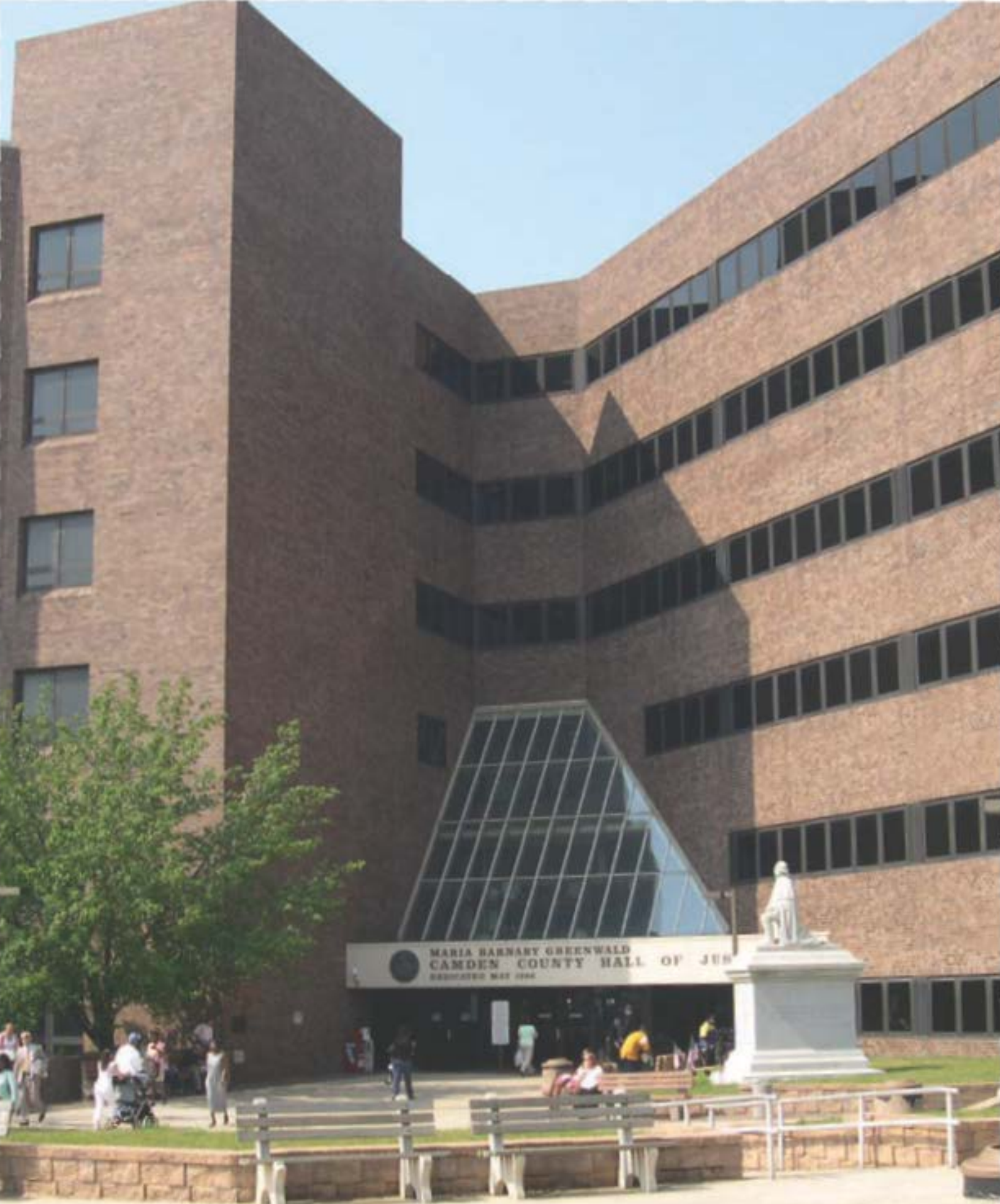
Camden County Hall of Justice
